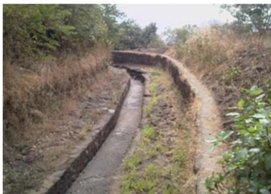
Fig. 5. Typical catch water drain on steep western slope.
